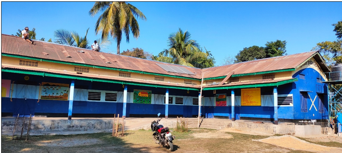
Figure 12: One of the schools with solar panels installed on the rooftop
